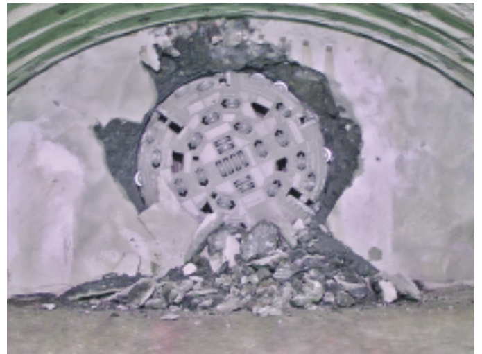
TBM施工状況
