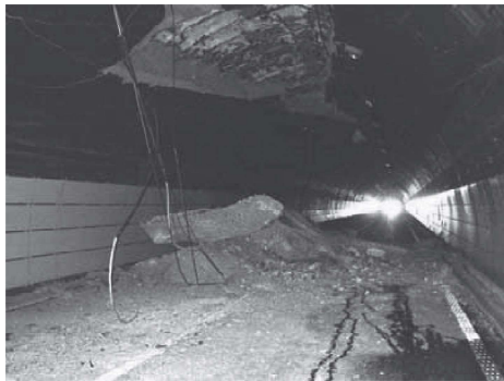
Photo 3. Damage of rock tunnel by Chuetsu Earthquake in 2004 (provided by MLIT Hokuriku Regional Development Bureau).
