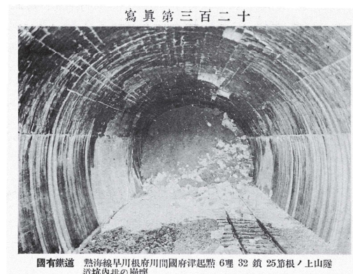
Photo 2. Damage of mountain tunnel by Kanto Earthquake in 1923 (from Digital archive of Japan Society of Civil Engineers, http://library.jsce.or.jp/Image_DB/shin-sai/kanto/jsce_report/jsccrp_02_04.html ).
