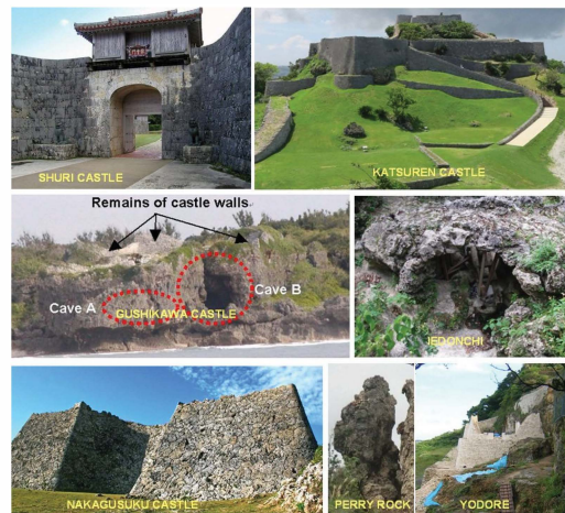
Figure 1. Some of historical masonry structures in Okinawa Island.
