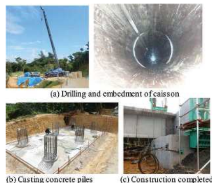
Figure 20. Stages of construction of piles and the bridge.
