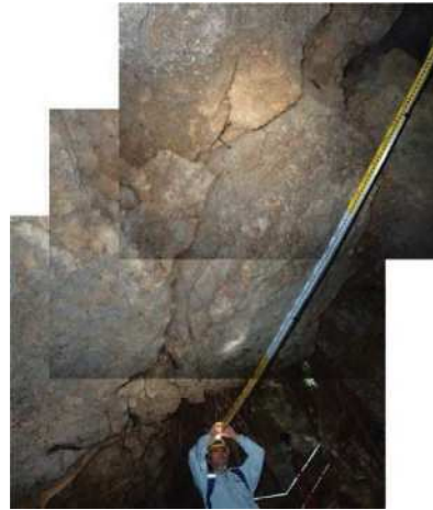
Figure 4. Status of the crown of the cave near exit (Area 7), note the movable block.
