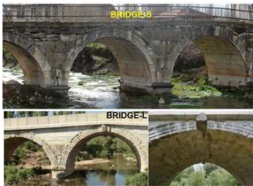
Figure 3. Relative separation and sliding observed in both bridges.
