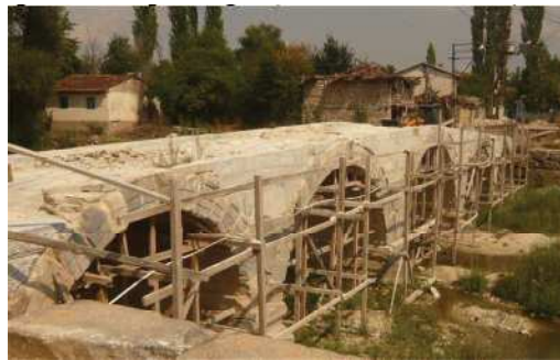
Figure 5. A view of Bridge-L after dismantling the asphalt pavement.
